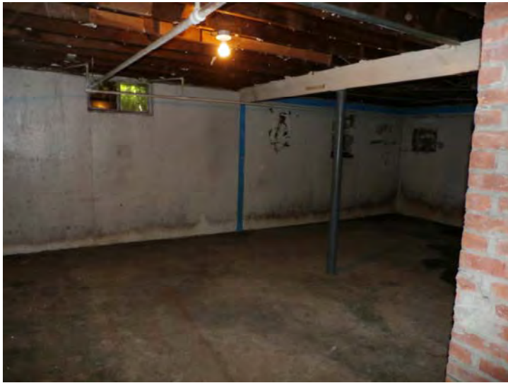
Typical basement area. Note water stain along wall
