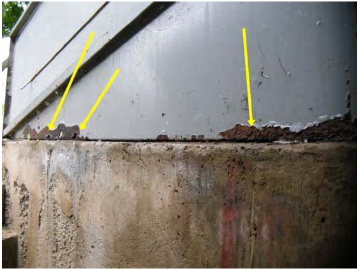
Typical bulkhead deterioration
