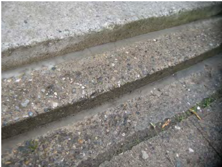
Typical example of concrete age related deterioration
