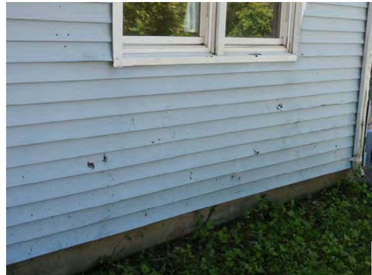
Example of common vinyl siding damage
