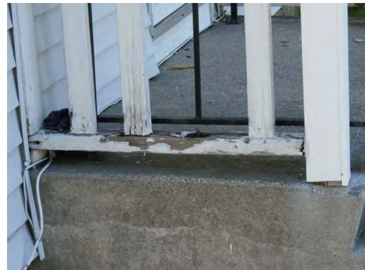
Example of porch deterioration
