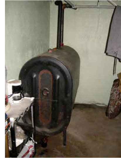
Typical fuel oil storage tank
