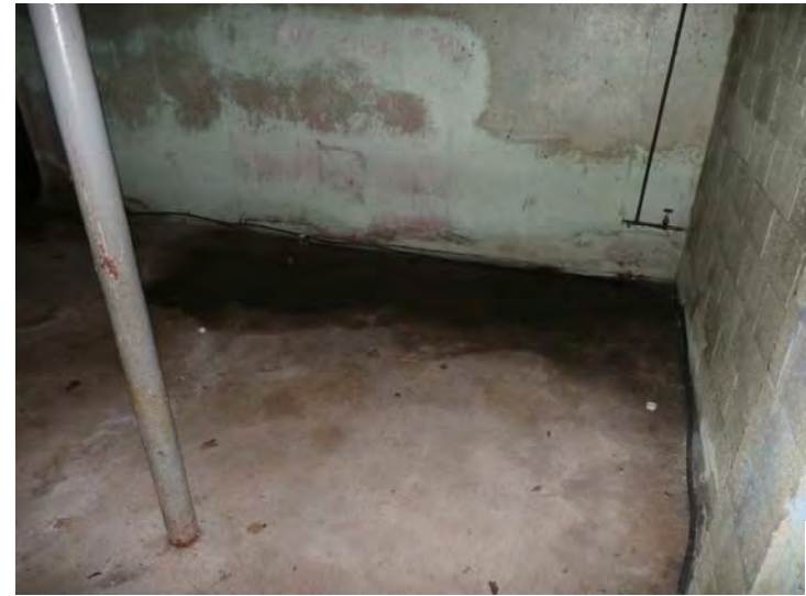
Typical example of basement water infiltration
